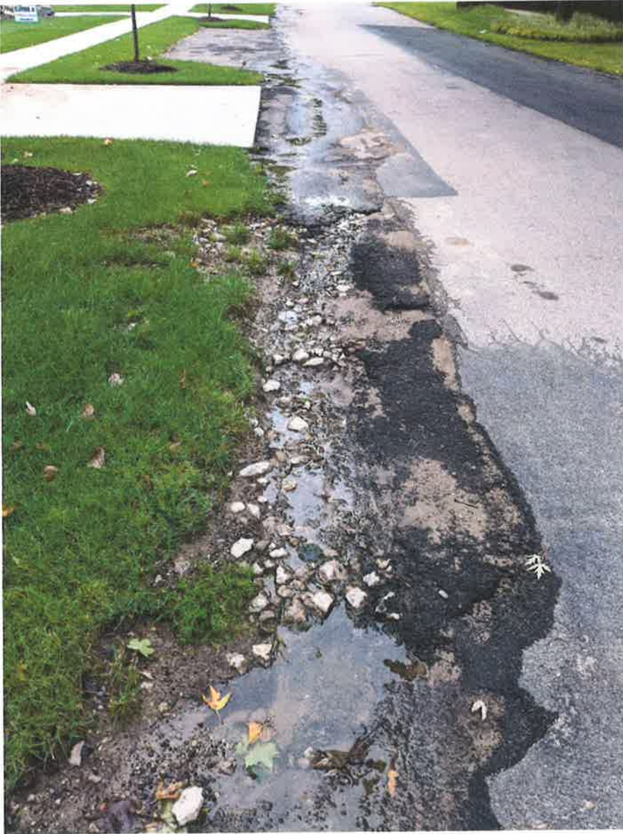
Picture 2: Pilgrim Ave erosion due to fast moving water/pooling
